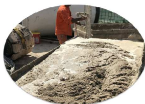
Soil conditioned with foaming agent
